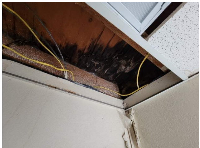
VIEW OF THE EXISTING ROOF DECK AT THE 1975 ADDITION
