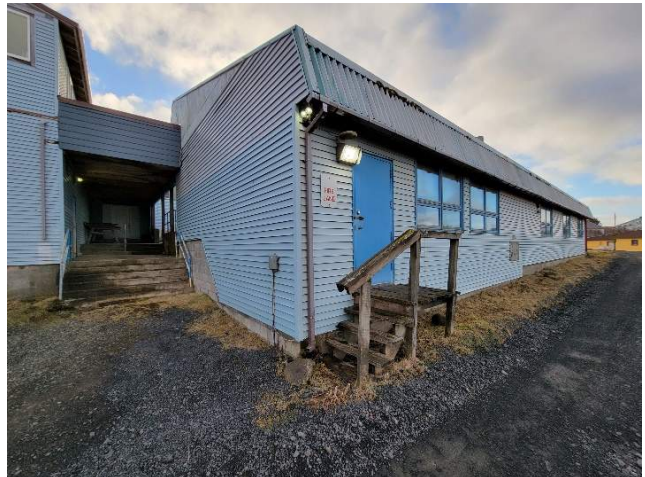
VIEW OF THE EXTERIOR EGRESS LANDINGS
