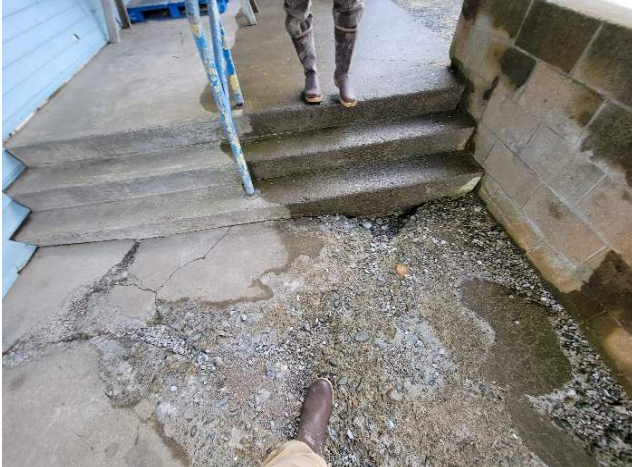
SIDEWALKS AT 1971 ADDITION
