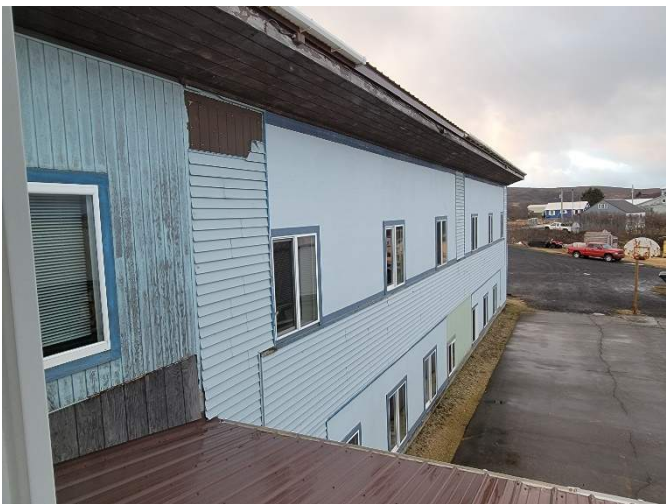
EXISTING SIDING AT THE TRANSITION OF THE ORIGINAL SCHOOL AND GYMNASIUM
