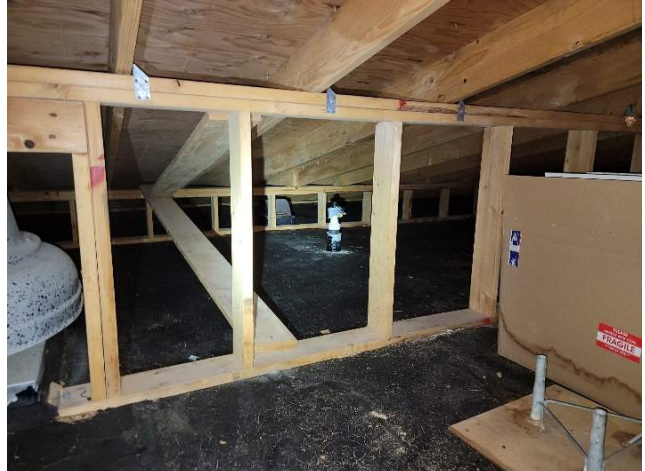
VENTED ROOF ATTIC SPACE WITH ORIGINAL ROOF BELOW
