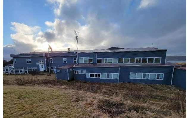
OVERALL VIEW FROM THE ADJACENT ROADWAY
