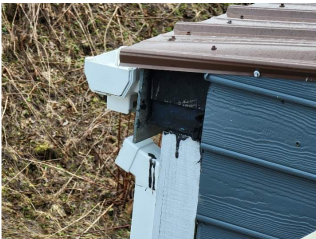
EXISTING GUTTERS AND ROOF SYSTEM
