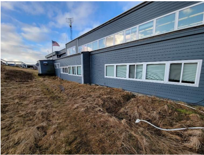
SITE CONDITION AT THE 1975 ADDITION
