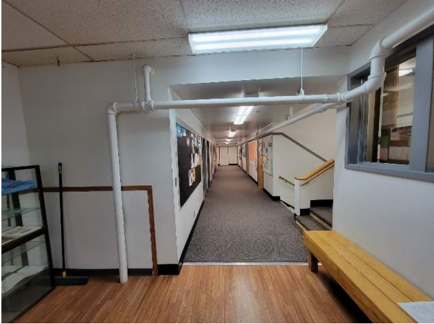
VIEW OF THE CORRIDOR AT THE 1975 ADDITION
