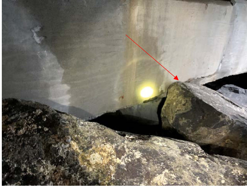
Figure 3: Abutment damage
