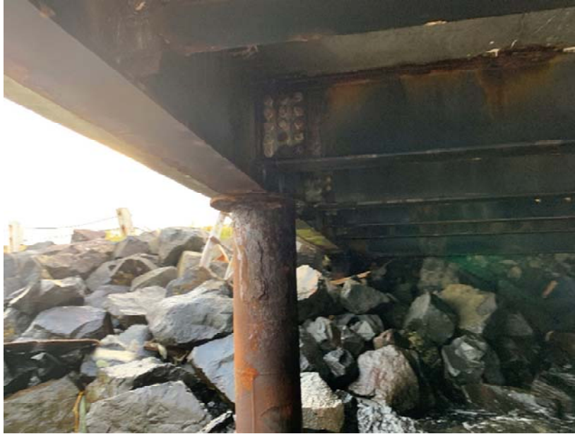
Figure 14: Typical pile condition, Pile B1
