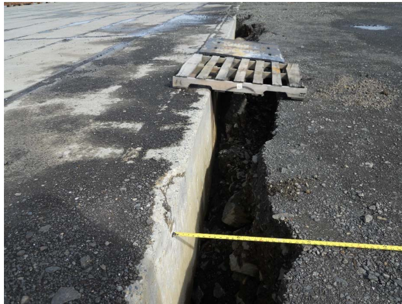
Figure 13: Fill settlement/separation
