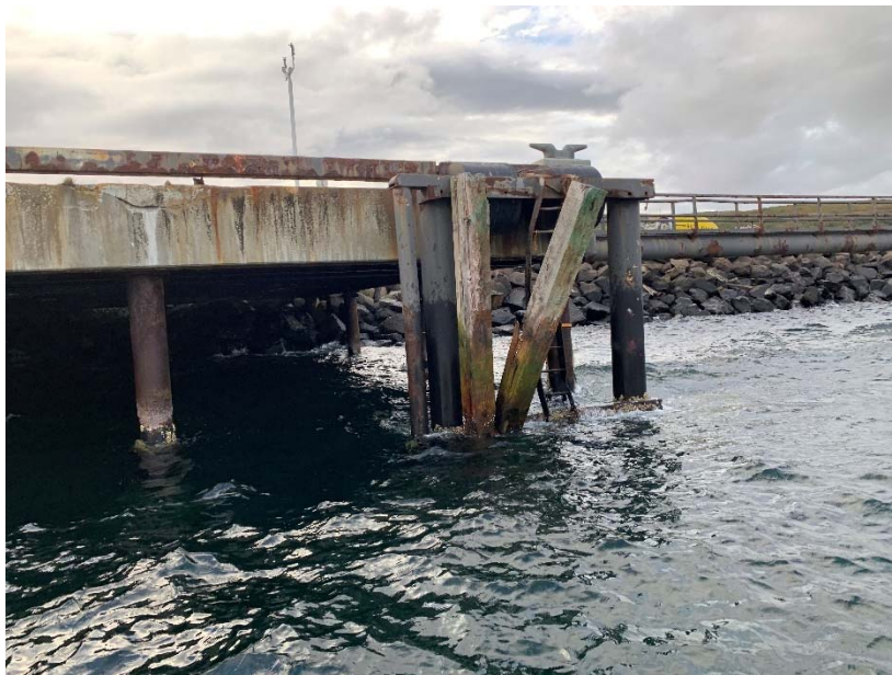
Figure 22: Damaged Timbers
